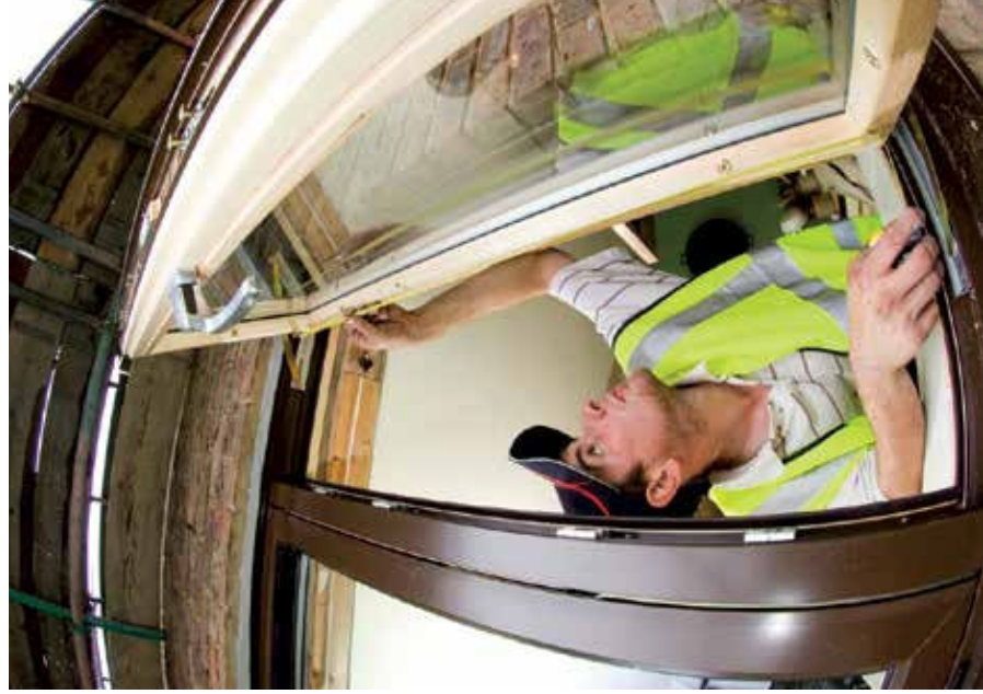
Repairs getting underway
